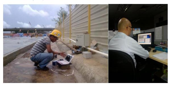
Before adopting I<sup>2</sup>R's technology, workers had to go on-site to about 40 times a week to manually retrieve data (left). After adopting the technology, workers are now able to access the data remotely from the office at regularly scheduled intervals (right).
