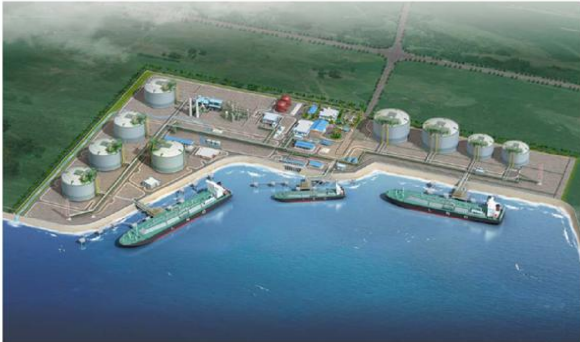
Artist Impression of the LNG Terminal with the Primary, Secondary and Tertiary Jetties
